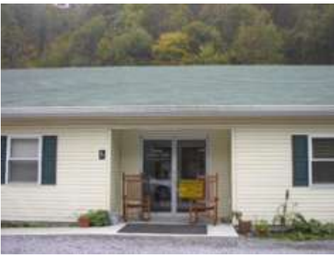
Highland Educational Project Facilities
